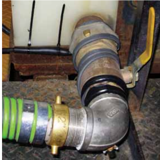
▲ Close-up showing the heater prior to wrapping with insulation
