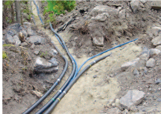
Installation of CARAPACE system.
